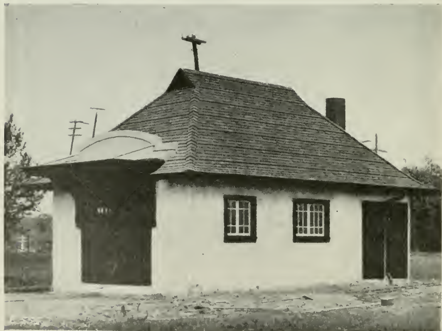
FIG. 50.—A GARAGE PARTIALLY BUILT OF CONCRETE.
